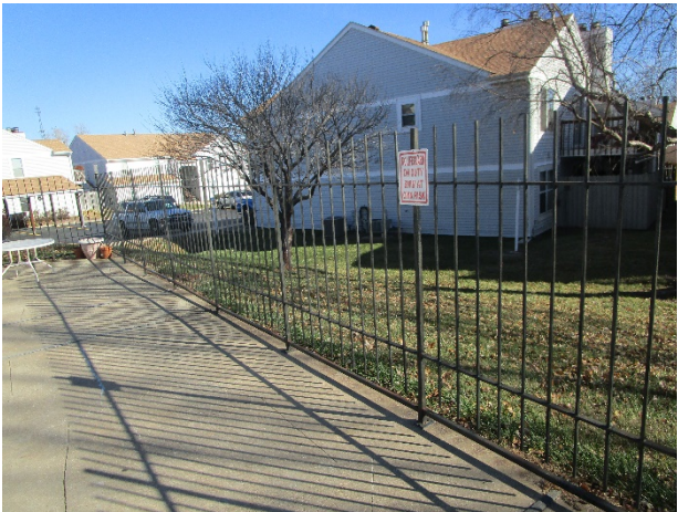
Metal pool fence overview
