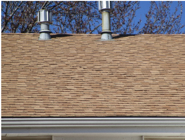
Shingle lift at Building 5851
