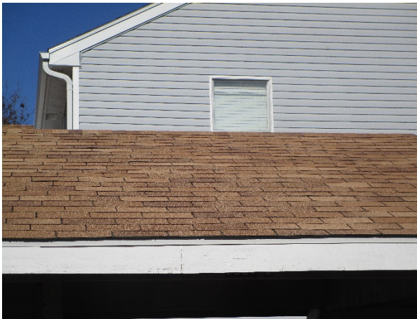
Shingle lift at the carport
