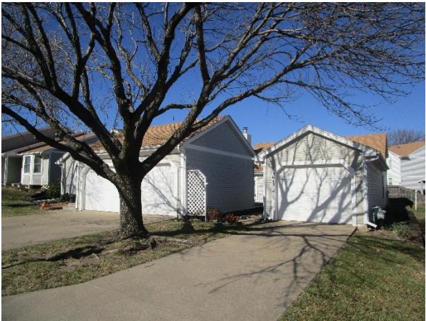
Concrete driveway overview
