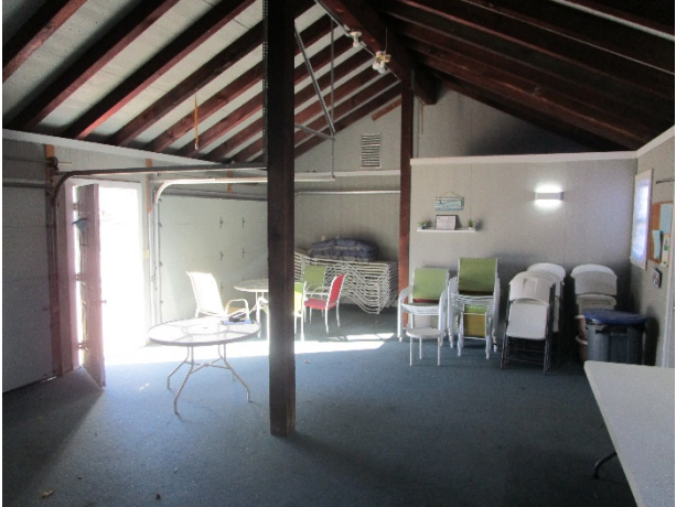
Pool house interior
