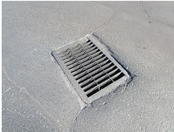
Catch basin overview
