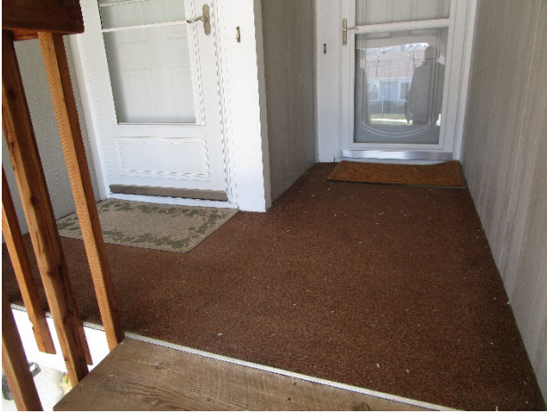
Staircase landing carpet floor covering
