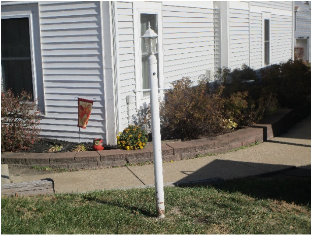
Light pole and fixture overview
