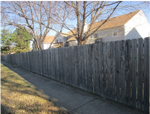
Front side of the wood perimeter fence
