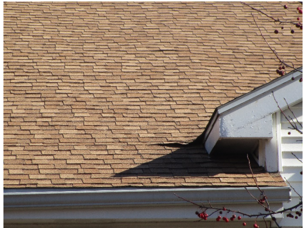
Shingle lift at Building 5811
