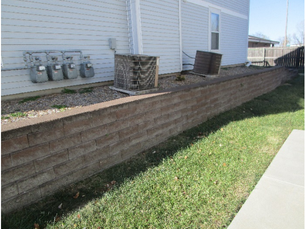
Masonry retaining wall
