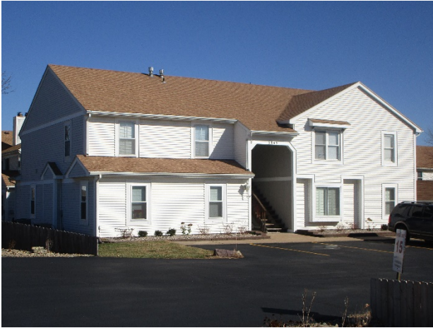
Asphalt shingle roof overview
