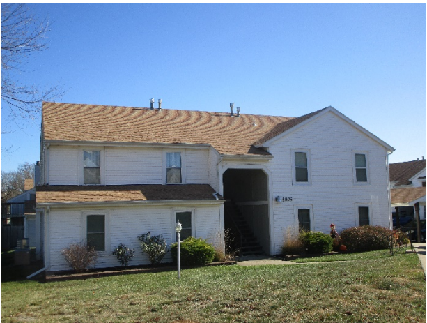
Apartment style fourplex front elevation
