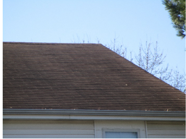
Shingle lift at Building 5859
