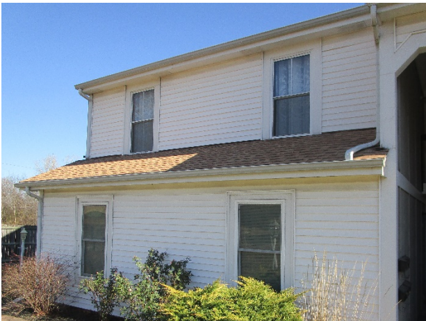
Gutter and downspout assembly
